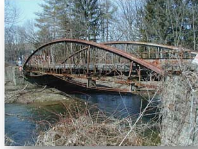
Ontelaunee Bridge Before the Move
