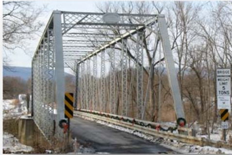
Neff Bridge Prior to Rehabilitation
