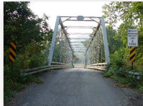
Neff Bridge After Rehabilitation
