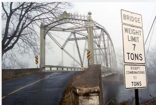
After the rehab!
