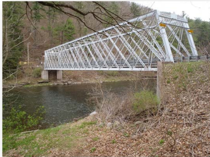
Upper Bridge at Slate Run
